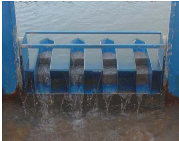
Fig.9. P.K.Weir with the outlet apron as steps
